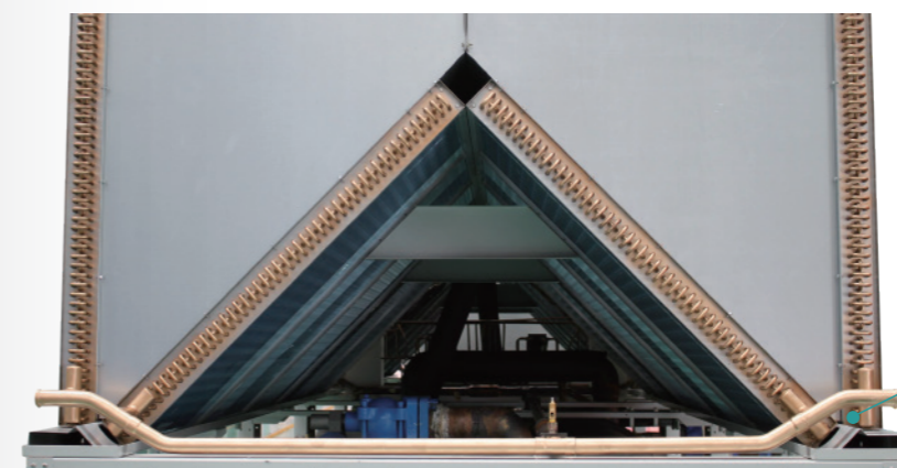
Special heat exchanger design for supercooling defrosting
